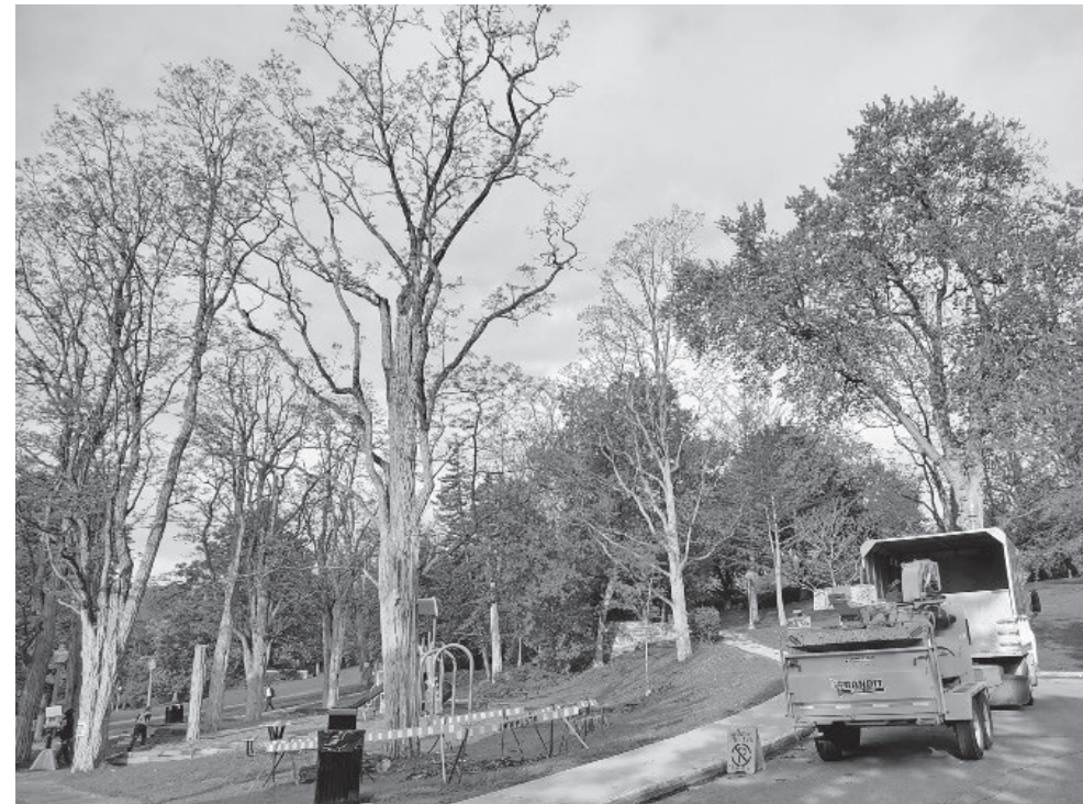
Work on the black locust trees in Murray Park has begun, as seen May 20. Some of the trees have been labelled green (for pruning), purple (for cabling/buttressing) and red (for removal). The grove reaches from mid-Murray Ave. to southeast of the field on Westmount Ave. For more history on the trees, including a photo from the 1920s or before, see March 27, 2018, p. RE-8.
